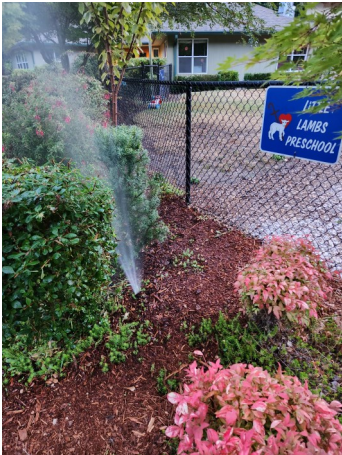
Sprinkler System Repair
