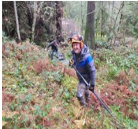
Brush Clearing at the Drain Field
